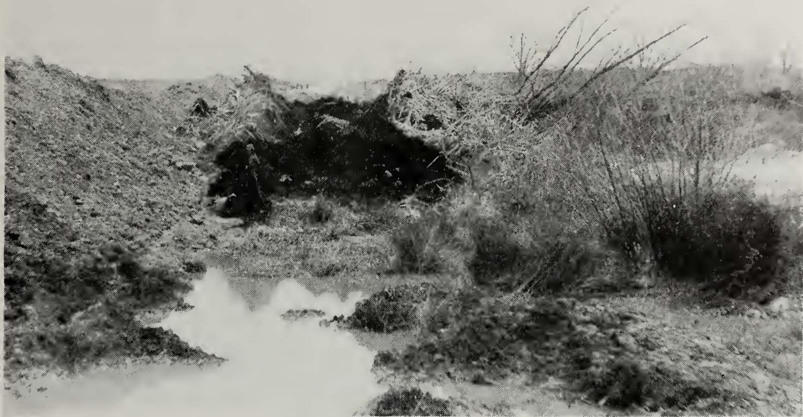
FIG. 23.—Muck and peat heaved by a highway fill across a swamp along 104th Avenue (Flavin Road) just south of 95th Street.
